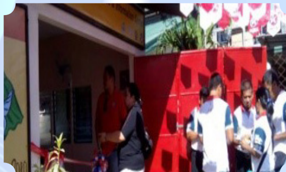
The Livelihood Enterprise Building of the Poro Sea Lovers Association in Barangay Poro with its officers and members
