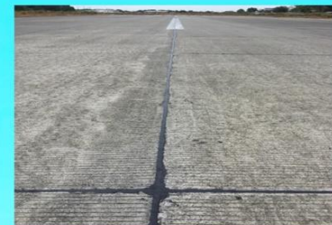
Application of Asphalt Sealant for the San Fernando Airport Runway
