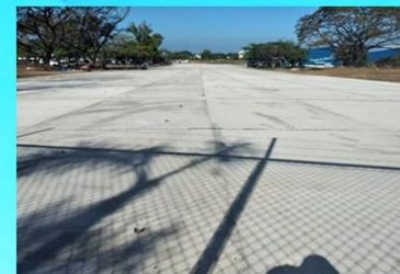
Construction of San Fernando Airport Access Road for Leasable Areas
