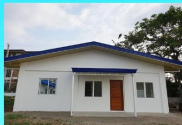
Rehabilitation of the CAAP Quarters with Proposed Expansion
