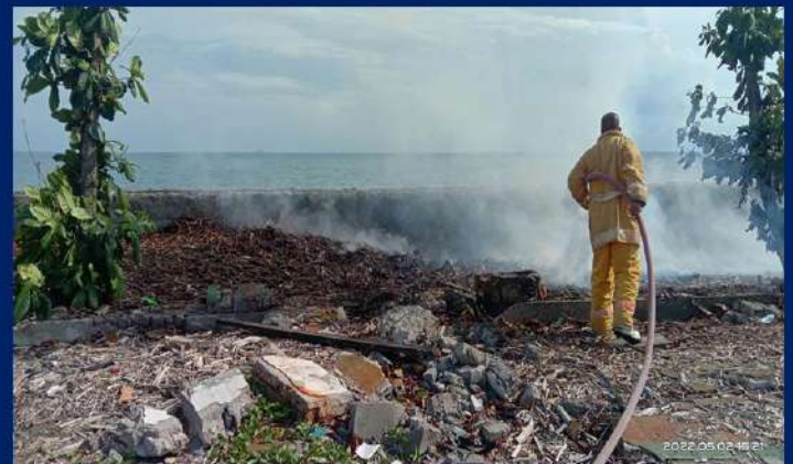
Responded demolition remains fire at Shippside area Poro Point.
