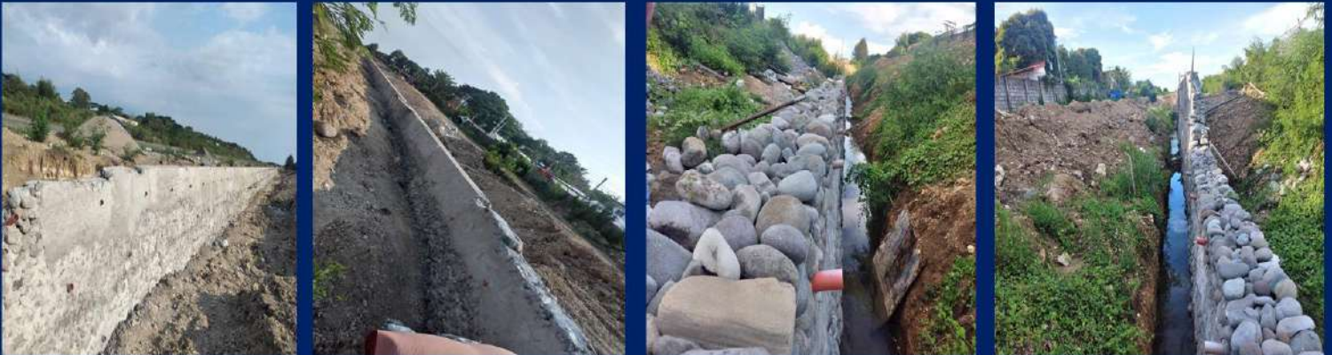
Construction of the San Fernando Airport Runway Slope Protection
